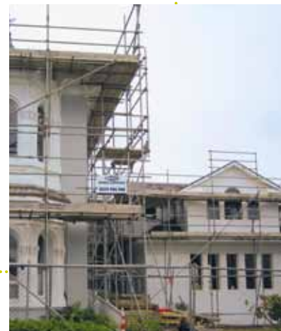
The Annexe, right, is to be replaced
