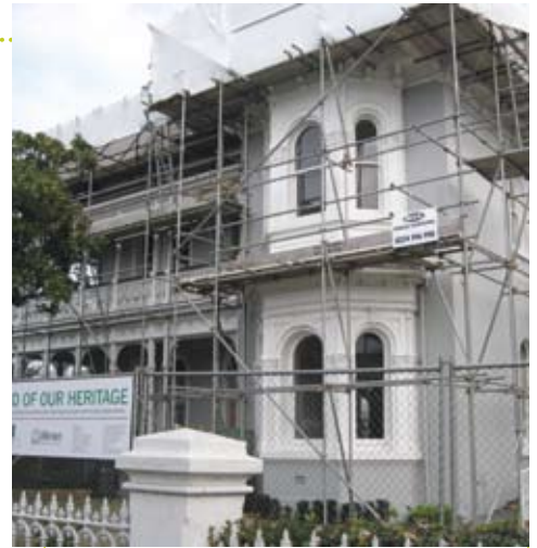
Allendale is still under wraps as renovations continue
