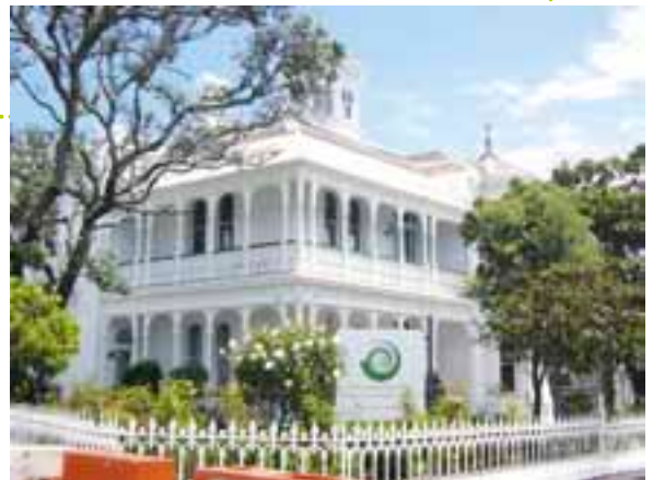
Essential repairs are planned for Allendale House
