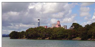
The refinery will still operate.
